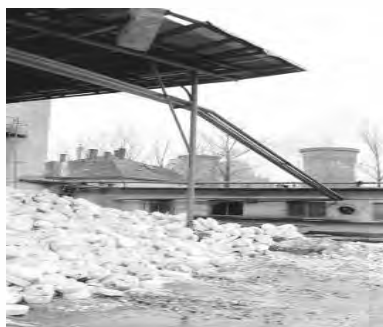
Figure 23.3. Storage of solids
