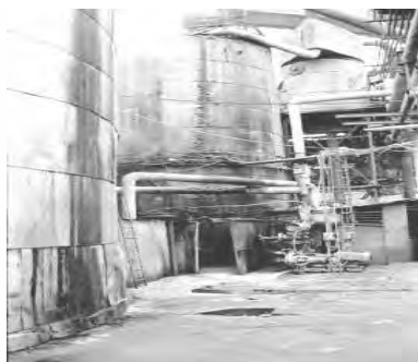
Figure 23.1. Leakages at a production plant
